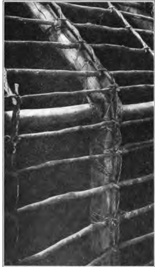
FIG. 82. JUNCTION OF RAFTER AND POST.
